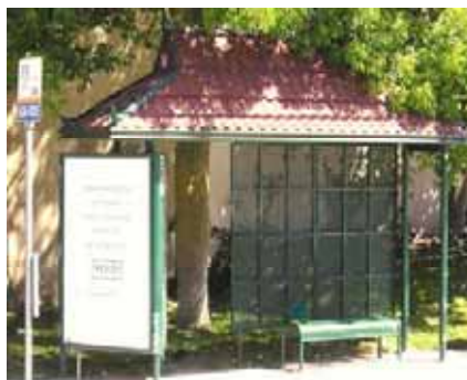
Westminster, CA bus shelter with a two sided kiosk at the end.
